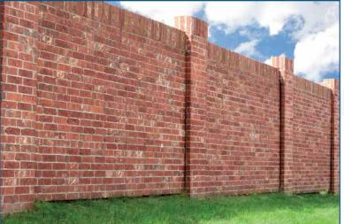
The "single wythe beam" panel supports itself without a continuous concrete foundation.
