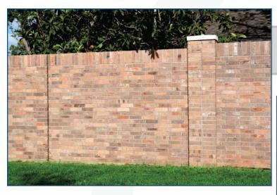
This method of installation allows each panel to move with the expansion of the surrounding soils which eliminates breaks and cracks in your fence.
