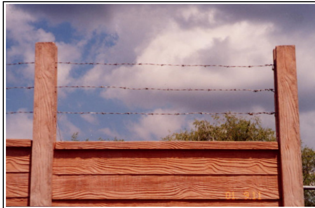
Wood Style Concrete Fence with Security Wire
