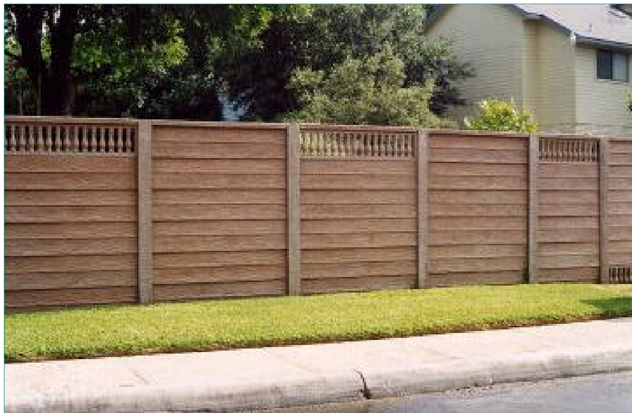
Wood Look Concrete Fence with Architectural Panels
